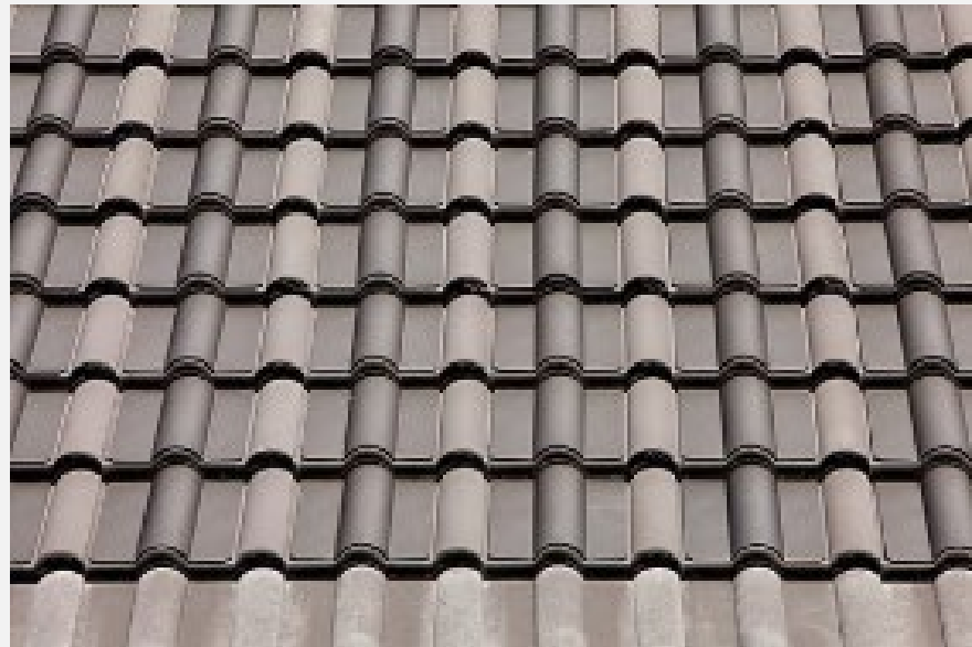
Roof made with solar roof collectors
